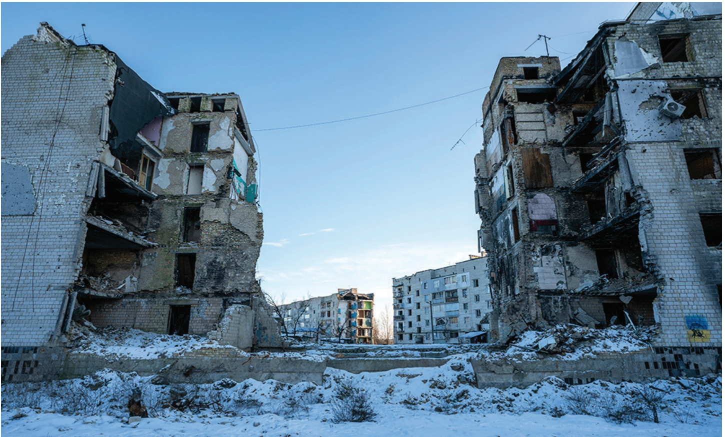
The center of this apartment complex in Borodyanka, Ukraine, collapsed when a Russian missile hit it on April 5, 2022. (Gregg Brekke)
