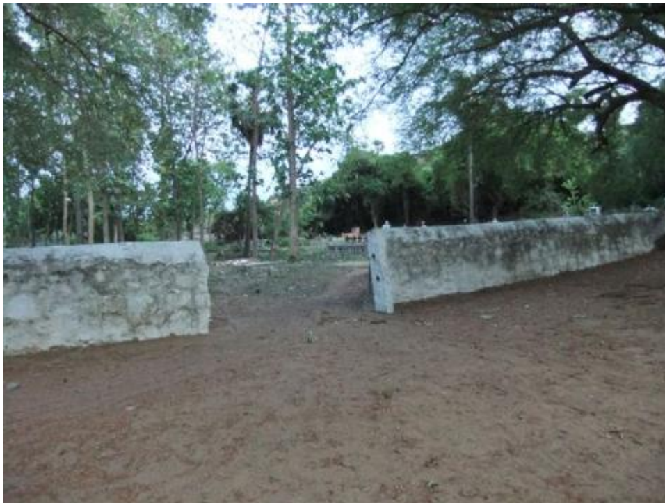
A wall divides Dalit and non-Dalit cemeteries on Catholic Church grounds in the southern Indian state of Tamil Nadu. (Courtesy of Robancy Amal Helen)
