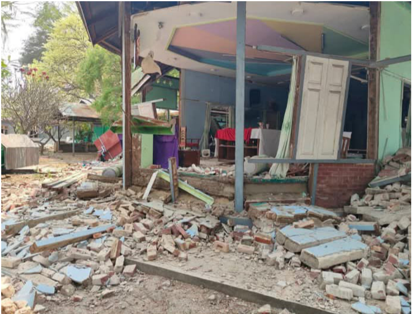
The front portion of the Mother of Sorrows convent in Mandalay, Myanmar, after the earthquake. (Courtesy of Josy Mary)
